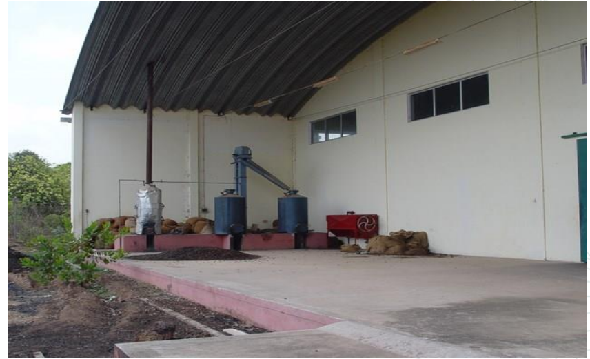
Cashew nut shell combustion plant, Guinea-Bissau
