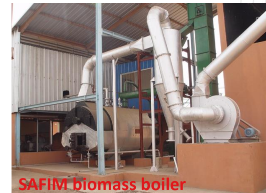
SAFIM power plant
