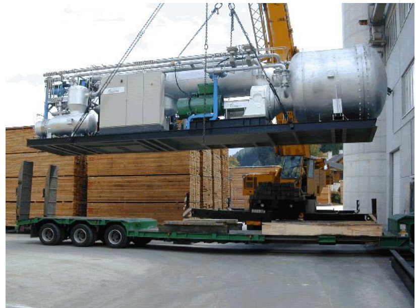
400 kW e ORC unit in Admont (Austria)
