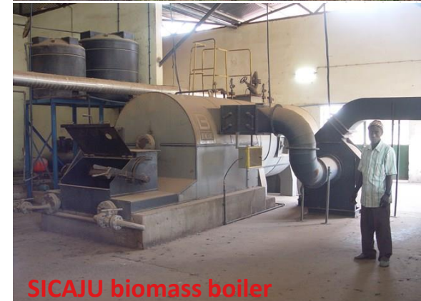
SICAJU power plant
