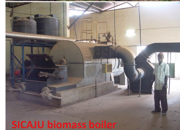
SICAJU power plant
