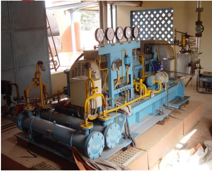
Steam turbine/alternator, Sicaju
