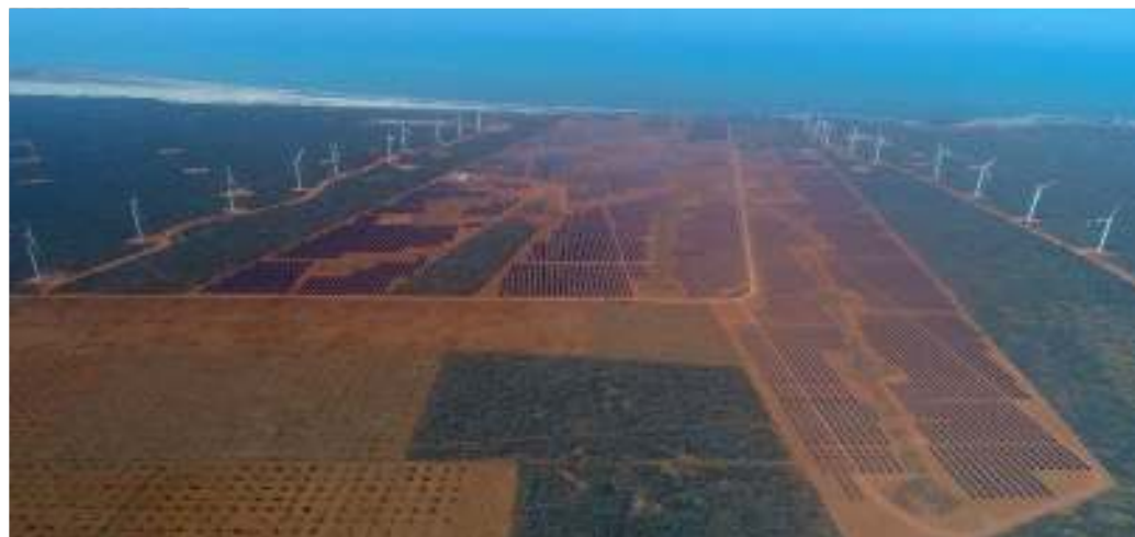
UFV de 101 MWp, Areia Branca (RN)
