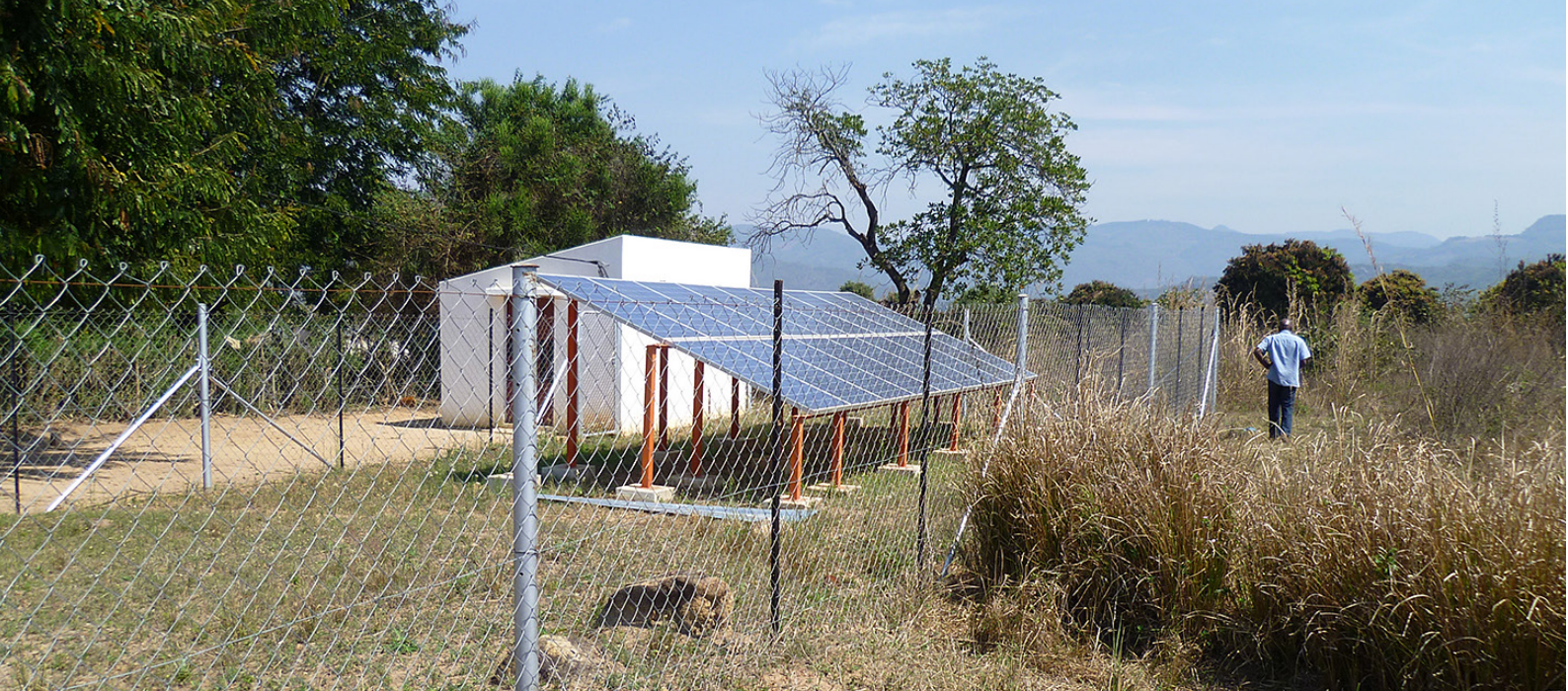
A solar mini-grid system in Chinhambuzi, Mozambique Source: Durham University, UK
