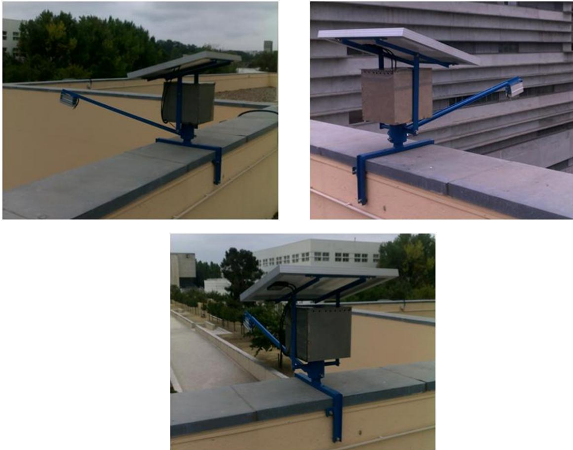
Figure 27 - Street lighting system installed at FCUL
