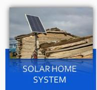
Stand-alone photovoltaic systems that offer a cost-effective means of supplying power for lighting and appliances to remote off-grid households
