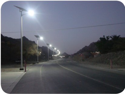
Solar street lighting
