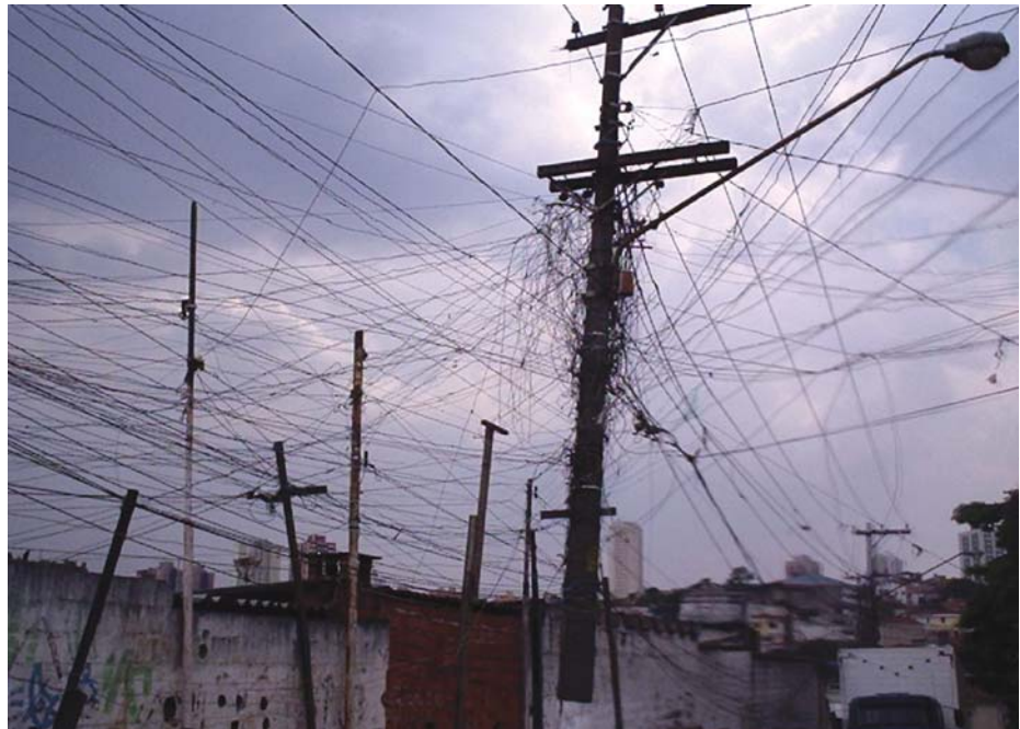
Type of illegal and unsafe connections that plagued a Brazilian utility before their successful intervention to prevent theft (Credit: Hans de Keulenaer)
