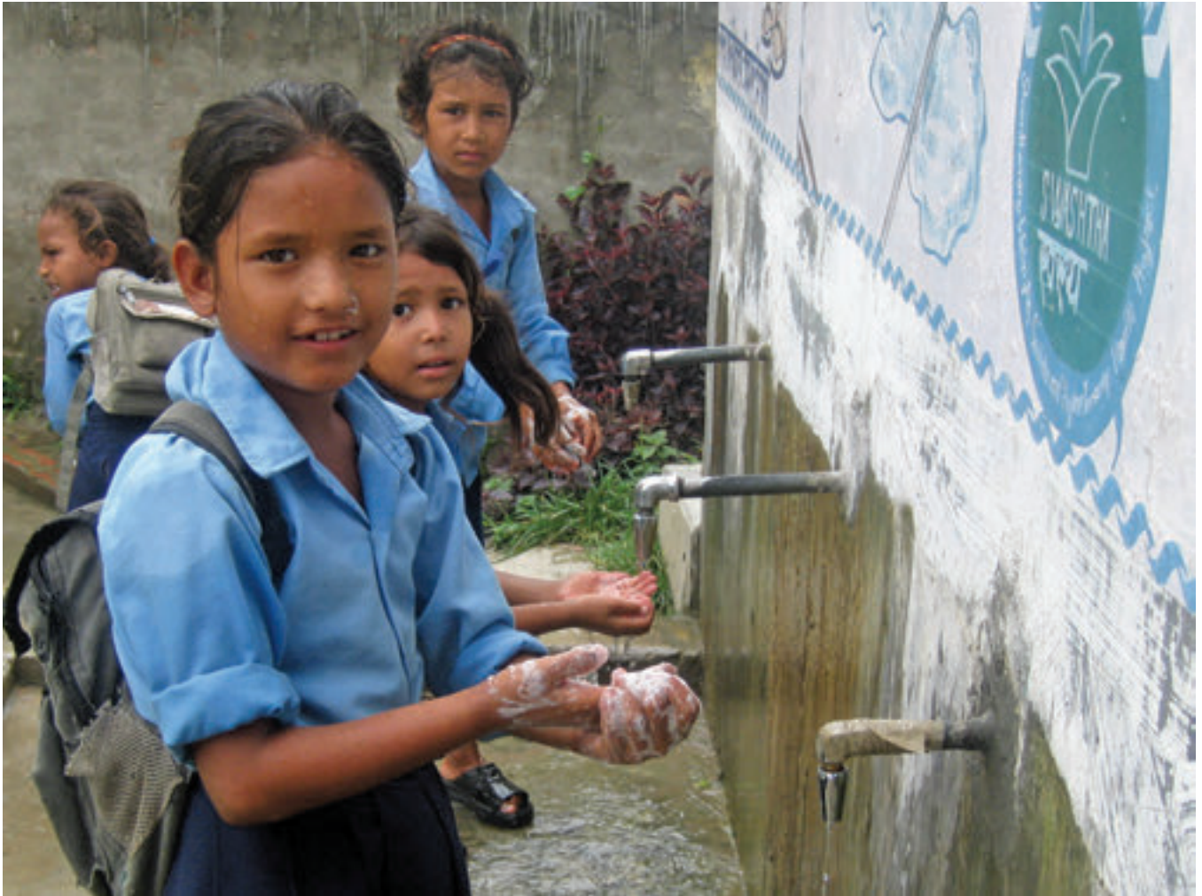
School children benefit from hand washing facilities in western Nepal. Water is provided from two types of storage tank, one which stores ground water pumped using grid electricity and another which stores water directly from a centrally piped distribution system (Practical Action Nepal)
