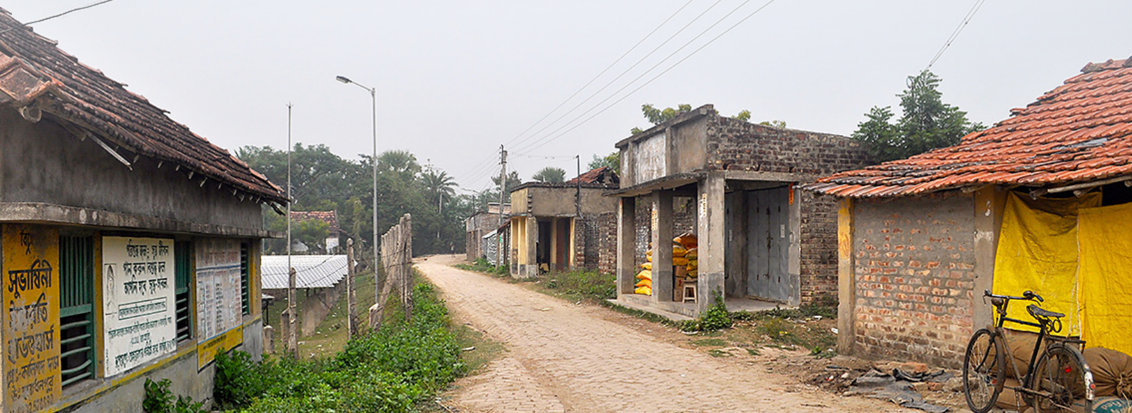
A street with distribution lines at a WBREDA microgrid site on Sagar Island, India.
