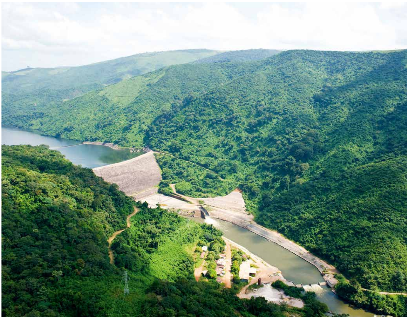
Hydropower Project, Sierra Leone.
