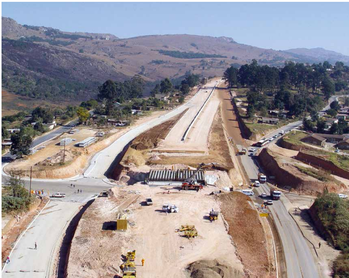
Investment in climate-resilient road infrastructure, Zambia.
