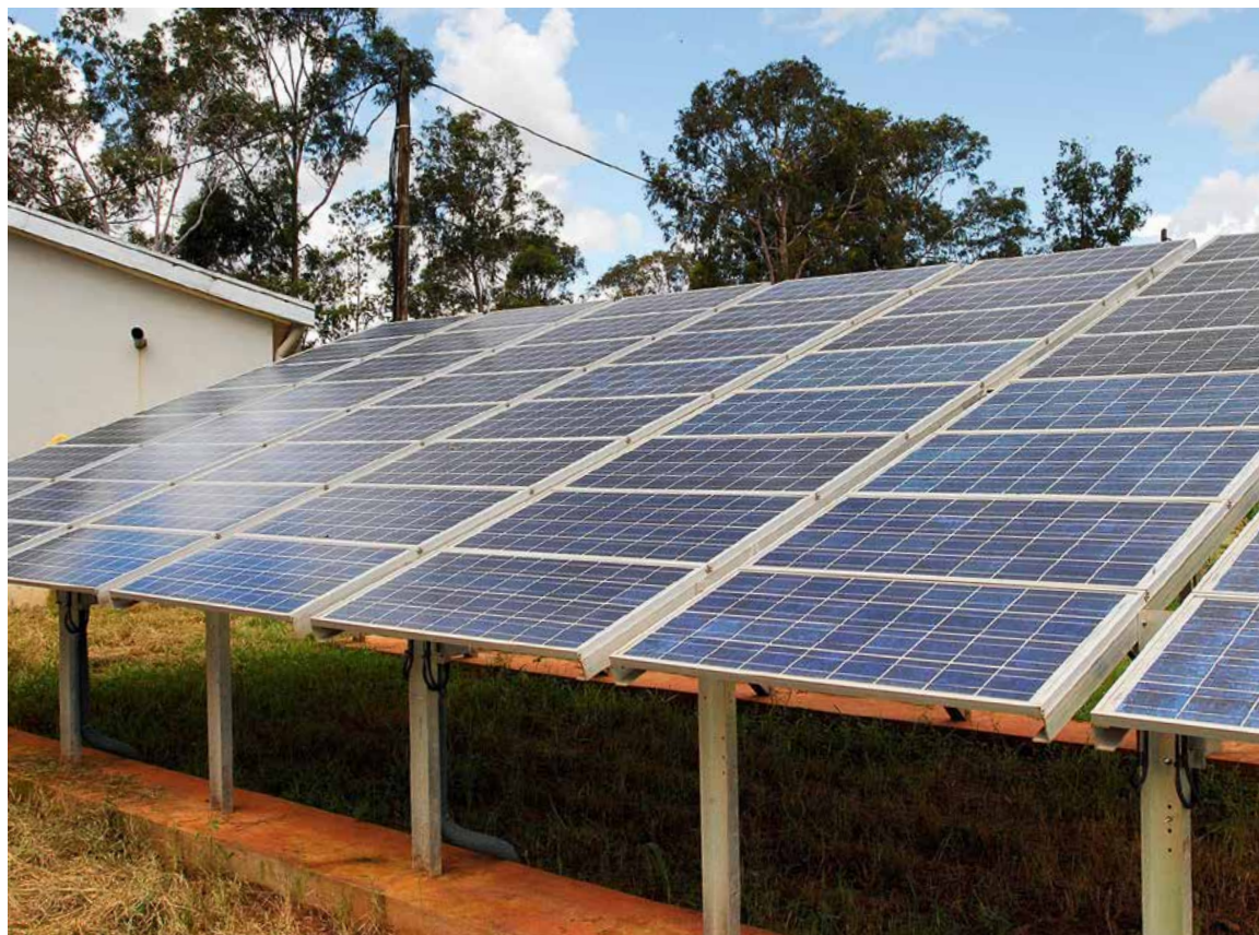
Solar Panel Electricity Generation, Madagascar.
