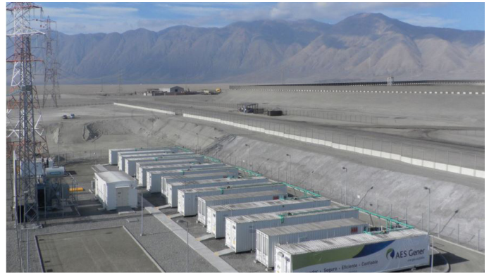
Picture 4.1 Lithium Ion Battery Containers at the AES Angamos Plant in Chile
