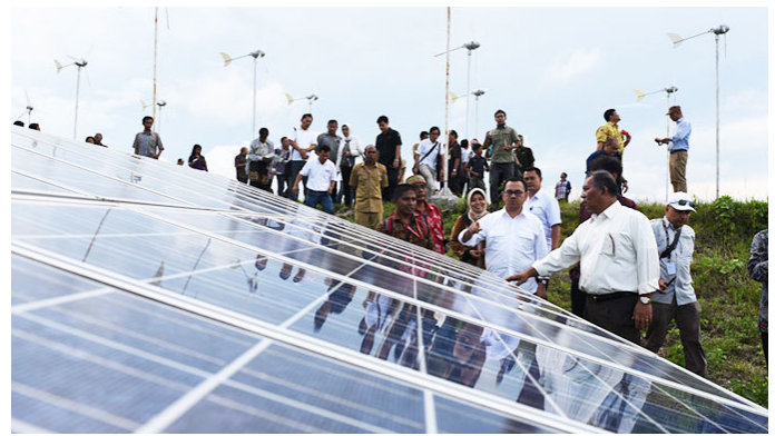
Picture 4.2 Commissioning Solar PV alongside Wind Farms on Sumba Island
