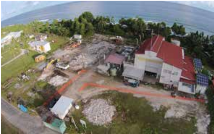
Pre-construction (diesel power station site)
