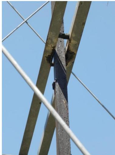
**Figure 54: (left) Windmill water pumping system in Mubalo and (right) wearing of the moving parts**
