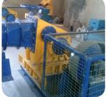
Service: Installation of Unido/Naseni (National Agency for Science and Engineering Infrastructure) fabricated crossflow turbines for electricity generation to provide reliable power to Ikeji-Ile-Ijesha, State of Osun, Nigeria. System: Cross-flow turbines for off-grid power generation. Generation: 70 kW
